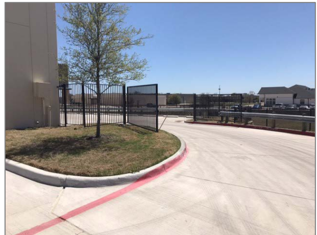
FIGURE 1: FENCE AND GATE
